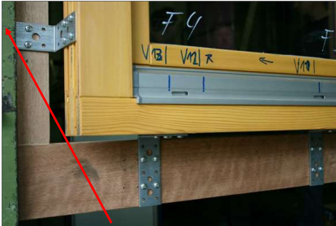
Detail Winkelbefestigung/ Bracket fastening detail
